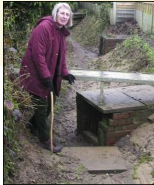
Cllr. Liz Robinson inspects the drainage ditch that was flooded, at the rear of properties in Valley Drive.
